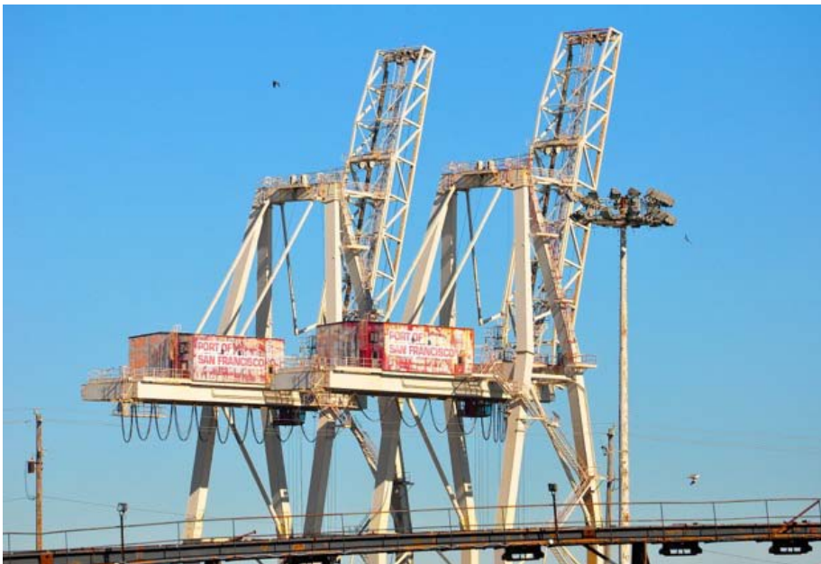
Port of San Francisco cranes nearby.
